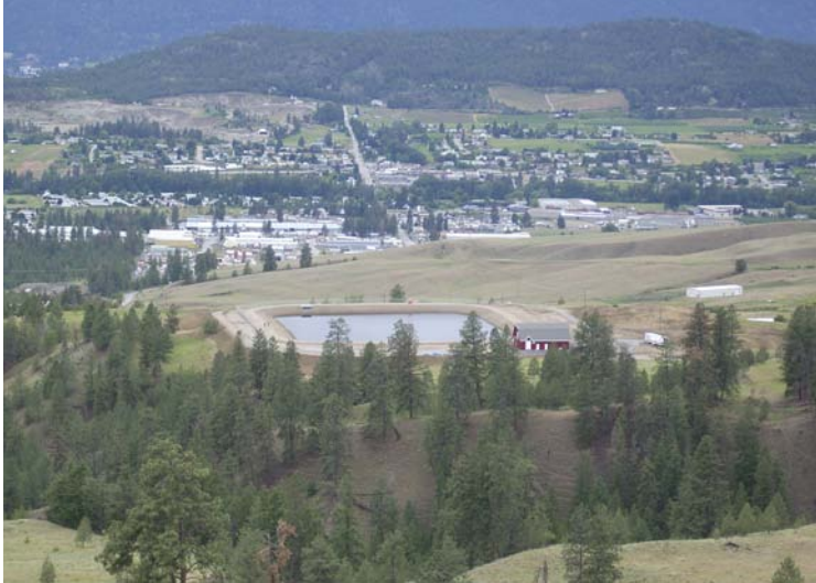
Lake Country's micro-hydroelectric generation plant will break the pressure of water as it enters this reservoir and simultaneously generate electricity (Photo: District of Lake Country).
