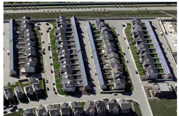
Drake Landing solar collectors (Photo: Natural Resources Canada/Doug McClenahan)
