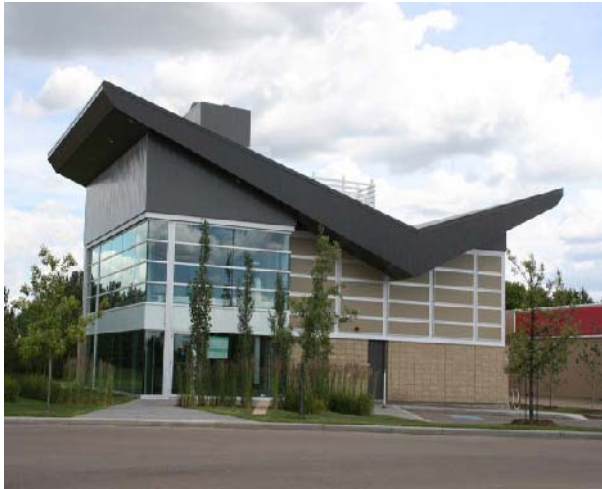
Strathcona County's Energy Centre (Photo: Strathcona County/Dwayne Welsh)
