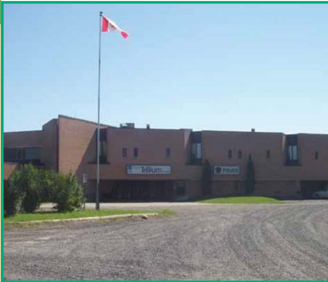
The former Trillium Centre in Sudbury, now the Lionel E. Lalonde Centre, incorporates recommendations from the energy audit.
